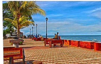
The shoreline of Culasi after the construction of the Seawall
